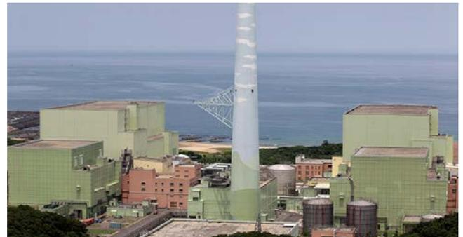
The Lungmen Nuclear Power Plant is a nuclear power plant in New Taipei City, Taiwan. It consists of two ABWRs each of 1,300 MWe net. It is owned by Taiwan Power Company (Taipower).
